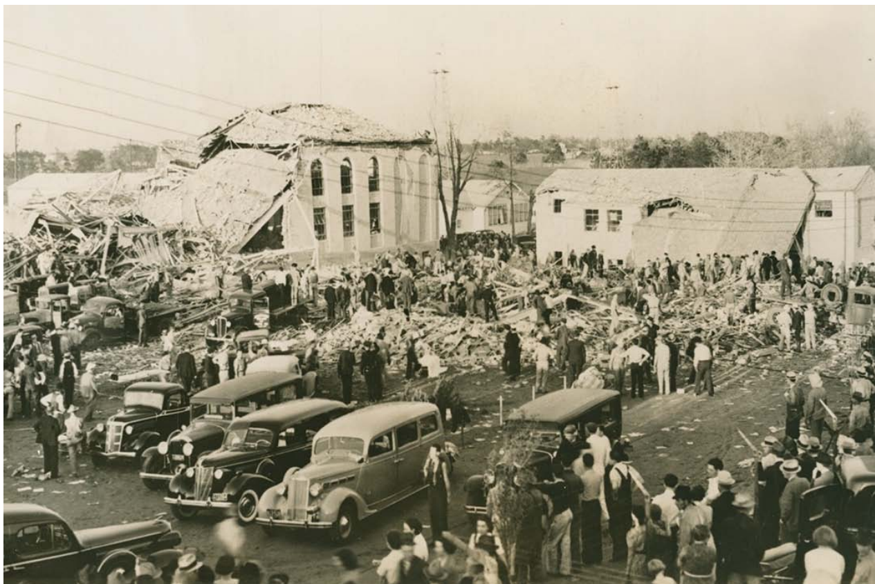
Remains of New London's school after 1937 gas explosion killed almost 300 people. Image source: Photo Archives cited in Texas Co-op Power Jan. 2017.
