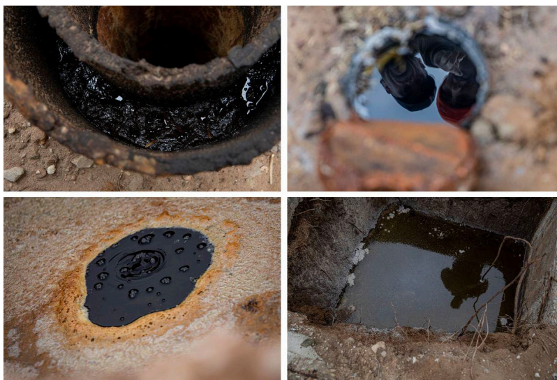
Figure 4. Various Leaks from Wells on Antina Ranch 39
